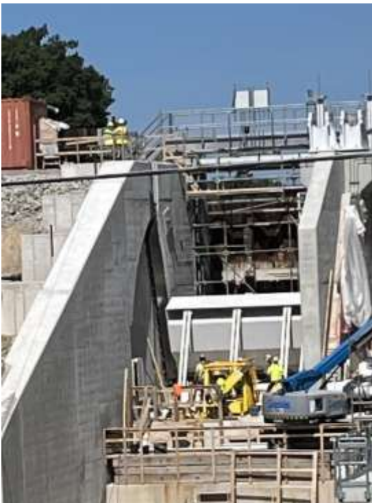
Photo From MONDAY, SEPT 14 th Installation Resumes of GATE 2
