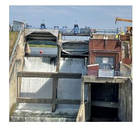
**Secord Gate Closure** - FLTF is closing one of the two gates at Secord Dam on a temporary basis for work on the low-level intake structure. The lake is not being refilled and little change in Secord Lake level is expected. This gate will be closed for periods of time over the next several weeks while stop-logs are installed to enable work to be completed safely. The gate will be returned to its fully opened position after the work.
